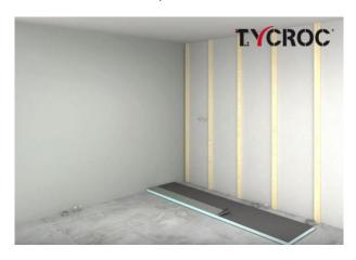
Apply the tiling compound evenly on the whole surface ot on the Tycroc TWP building board. Press the board against the wall and level
