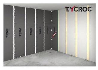
Direct water contacted corners, cover additionally with waterproofing tape and -membrane.
