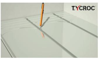
For a U-turn or crossing channels near the walls, cut the aluminium foil with a knife first to "open" the channels, and press the foil into the channel, using e.g. a knife handle.
