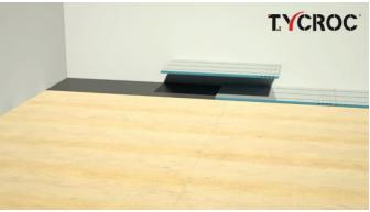
Place the panels onto the mixture and press down lightly. Check that the panels are levelled on the floor (as a good tool for levelling, a hammer and a wooden support board or block can be used – level the panel to its place by tapping).
