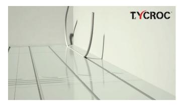
Press the floor heating pipe by hand or foot into the Tycroc UHP channels. Ensure that the pipe reaches connection point and adding 1m.
