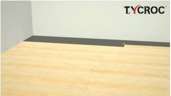
The underlying surface has to be free from dirt, oil or other lubricants and it cannot be frozen. Transfer the adhesive to the underlying surface (for better bonding, cover the surface prior to the gluing with adhesive dispersion).
