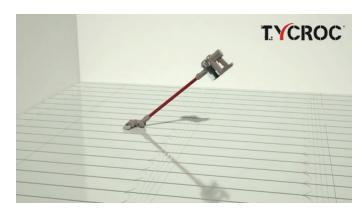
Before the installation of the heating pipe make sure that the channels are clean of dirt Avoid too many steps on the emty channels to not broke the edges of the channels
