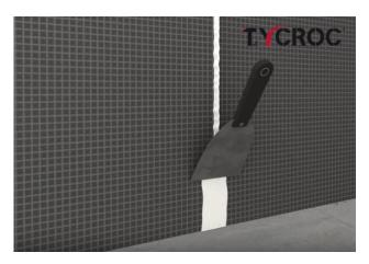
The gaps between building boards and corners should be covered with adhesive sealant, and also fastening washers should be covered with the help of a spittle. Direct water contacted corners, cover additionally with waterproofing tape and —membrane.
