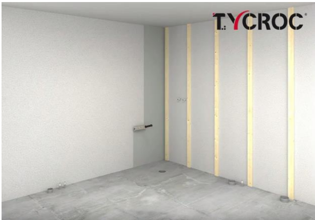
Apply primer component to the wall.
