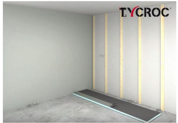
Apply the tiling compound evenly on the whole surface of the Tycroc TWP building board. Press the board against the wall and level.
