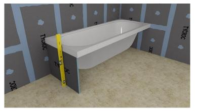
Apply similar line of the adhesive sealant to the board edge coming into contact with the rear wall. Thereafter, install the board to the intended place under the bath edge, then level and fasten it.
